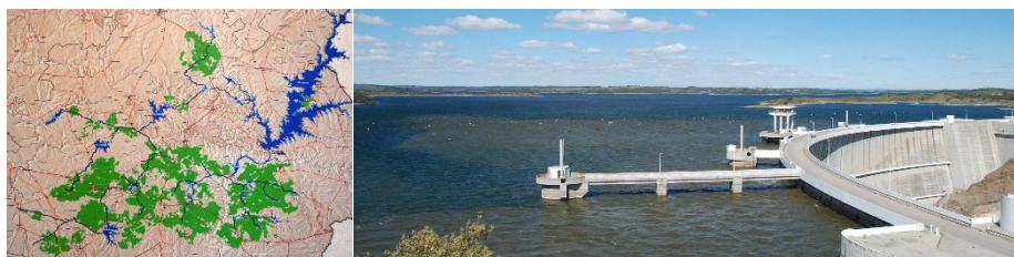
Figure 3. Alqueva hydroelectric dam (and its map with the effected areas) visited by the COST TU1401 RELY (Renewable Energy and Landscape Quality) participants on the 25 th of March, 2015
