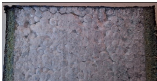
Fig. 5. Core failure morphology
