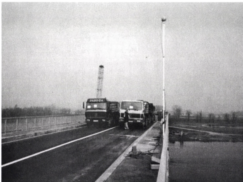
Fig. 3. Details in test loading and measuring of deformations
