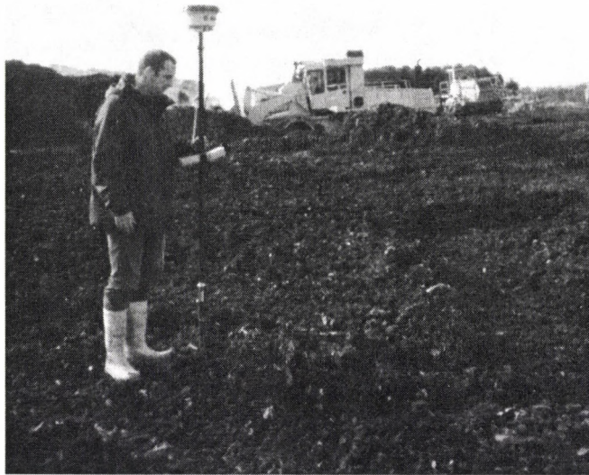
Fig. 1. RTK measurements on dumping ground (Rover)
