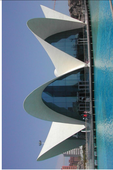
Steel fiber reinforced concrete thin shell structure Oceanographic Park Restaurant. City of Arts and Sciences, Valencia (2002) Based on blueprint of Felix Candela, by: A. Domingo, C. Lázaro, P. Serna
