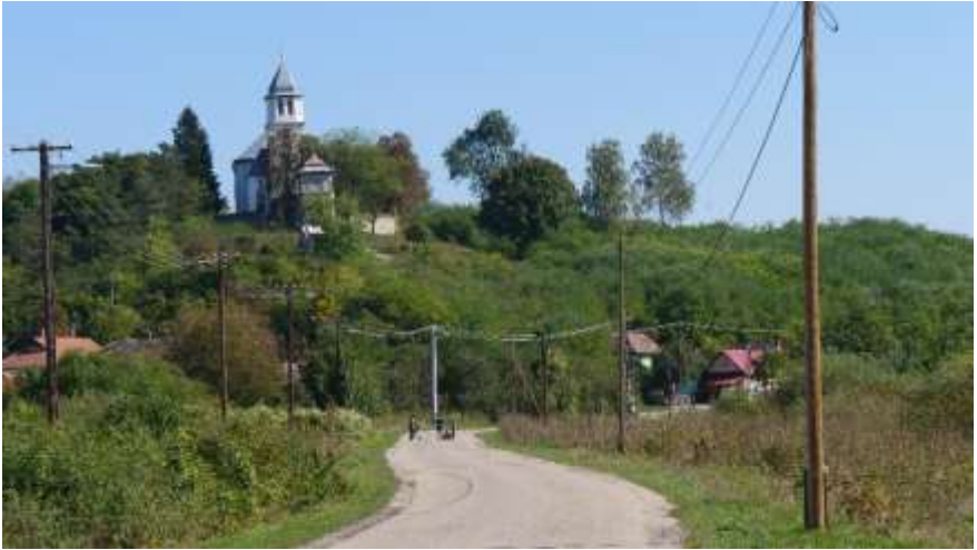
The Greek Catholic church in Rakaca, an exemplary maintained building, dominates the landscape.
