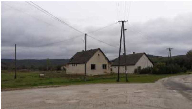
Figure 10. Abandoned houses at the edge of the village in Meszes
