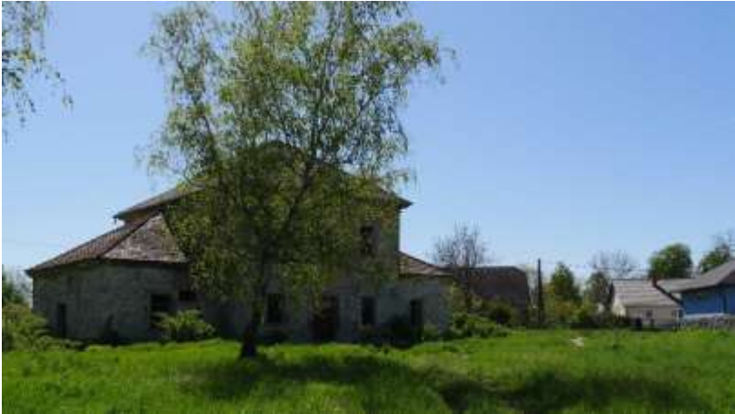
The ruined building of the Szathmáry Király Castle in Boldva.
