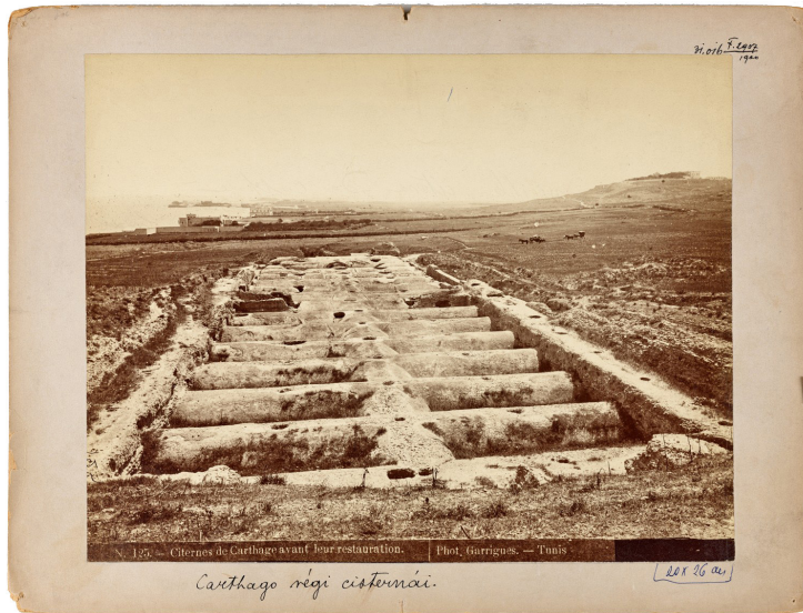
25. The cisterns of Carthage before their restoration. Tunisia, 1864–1884.
