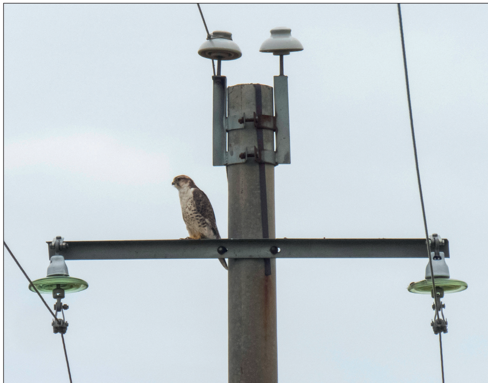
Figure 3. Saker Falcon perched at experimental pole with an additional unconnected pin-insulator fitted to P1 to deflect birds from dangerous perch sites at the concrete pole top, and suspended insulators to separate conductors at P2/3 from perch sites on crossarm
