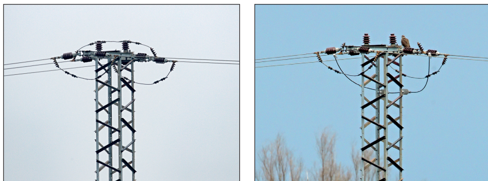
Figure 14. Dangerous jumper in upper position on a 22 kV tower (left) and change of its placement under the plane of main wires (right). Photo: J. Chavko
