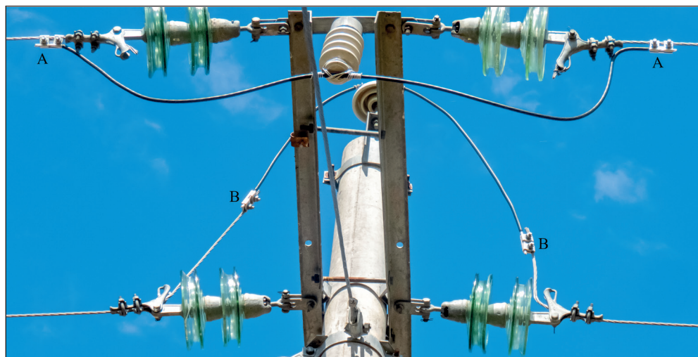
Figure 5. Insulated jumper wires connected to conductors at anchor pole. A: shows correct fitting at P2/3 with cable connection in front of the dead-end clamp. B: shows incorrect fitting at P1 with cable connection on jumper wire after the dead-clamp, leaving exposed conductors above perch sites on the crossarm
