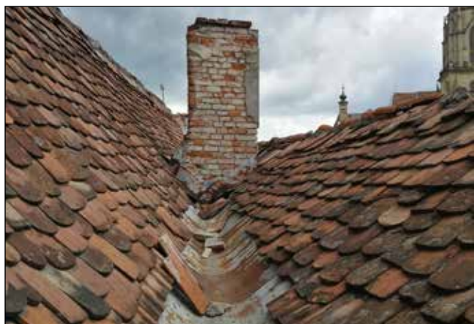
■ Fig. 8. Acoperiș „jgheab colector”. © Georgiana TIRT ■ Fig. 8. The “Rain gutter” roof. © Georgiana TIRT
