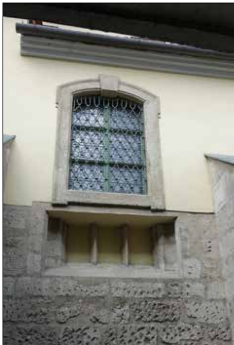
■ Fig. 10. Budapest, Biserica parohială Nagyboldogasszony, sub fereastra barocă au fost evidențiate profilele ferestrei anterioare gotice, iar piatra fătuită gotică a fost martelată pentru a suporta tencuiala barocă, acum eliminată de restauratori. © Virgil POP ■ Fig. 10. Budapest, Nagyboldogasszony Parish Church, under the Baroque window, the profiles of the previous Gothic window were highlighted, and the Gothic stone facing was hammered to support the Baroque plaster, now removed by conservationists. © Virgil POP
