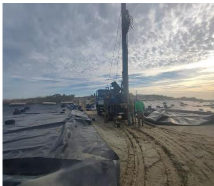
Figure 1. Field investigation (Drilling)
