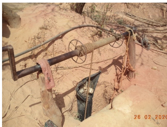
Figure 4. The well ventilation system using an agitation head.
