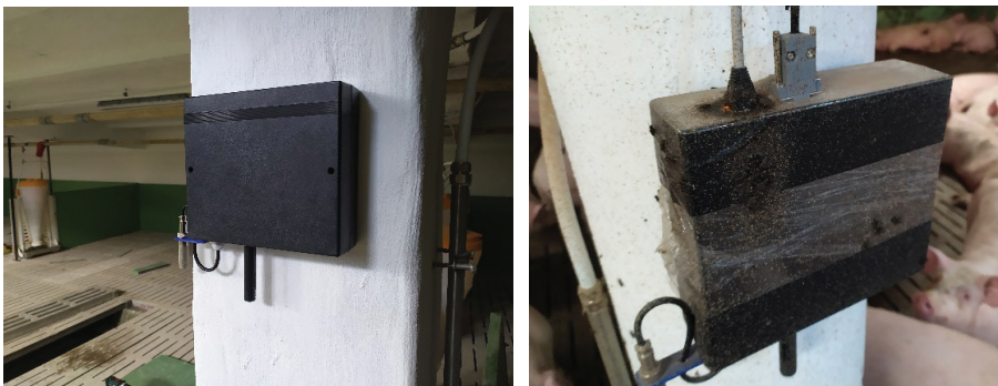
Figure 5. Boxed multisensor on site: fresh (left), later (right)
