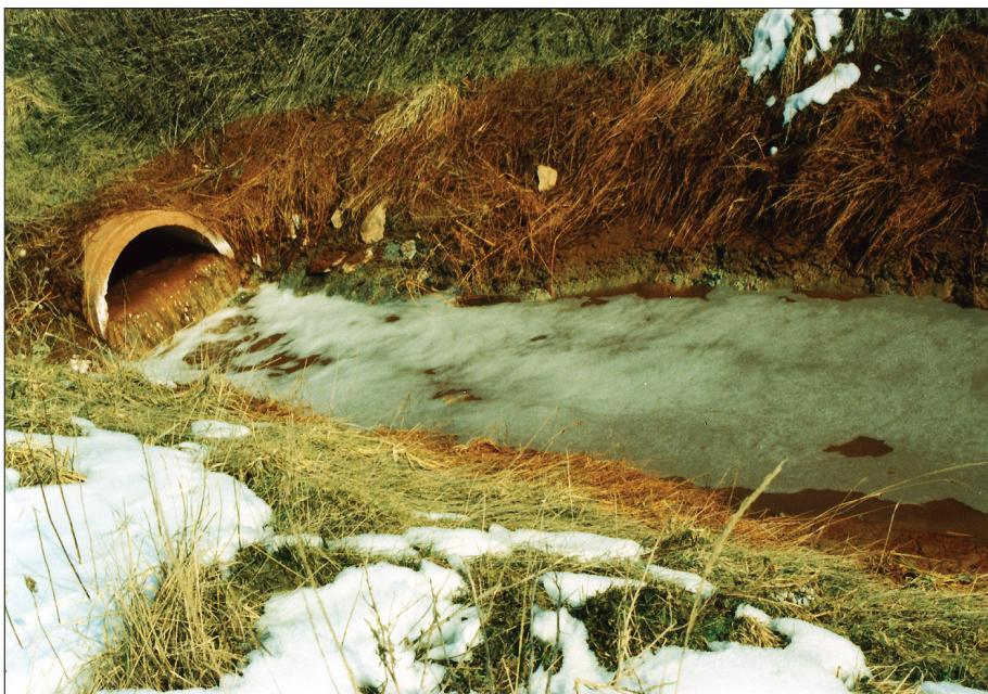
*Photo 2. Foamy alkaline water flowing out of leakage of sludge reservoir (Photo by JUHÁSZ, Á. 2003)*
