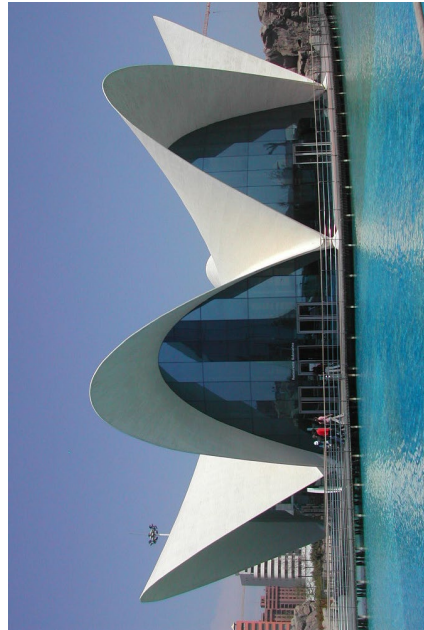
Steel fiber reinforced concrete thin shell structure Oceanographic Park Restaurant. City of Arts and Sciences , Valencia (2002) Based on blueprint of Felix Candela, by: A. Domingo, C. ) Lázaro, P. Seina
