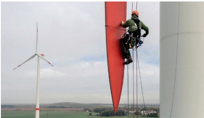
Figure 11. Application of rope technique [14]
