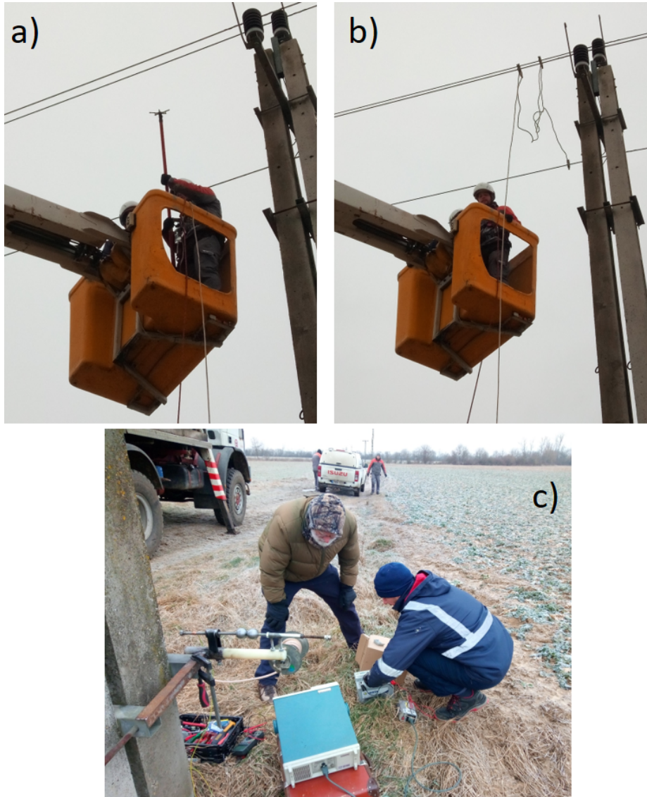
Fig. 5. Preparations at the first test location. (a) Testing for high voltage. (b) Combining the 3 wires (phases). (c) Dániel Piri (to the right) and professor Earle Williams are assembling the oscilloscope, inverter, and car battery. The spark gap (to the left) is fixed to the grounding of the pole and the reel of the down-coming cable from the combined line is already attached to its right side.
