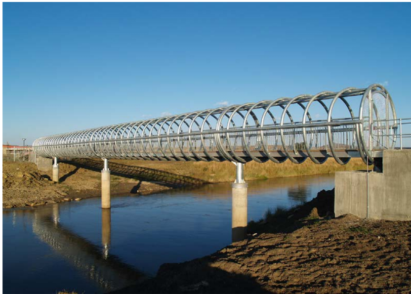
Figure 5. Ncome Museum Pedestrian Spiral Bridge
