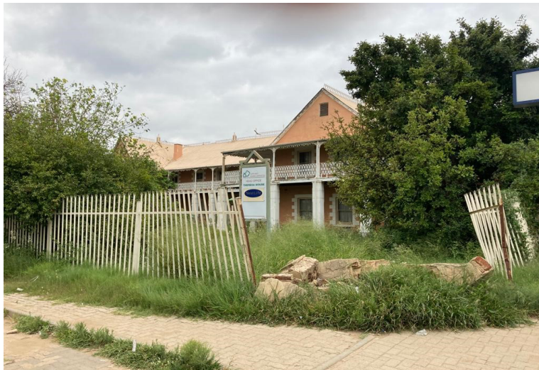
Figure 4. Theresa House neglect
