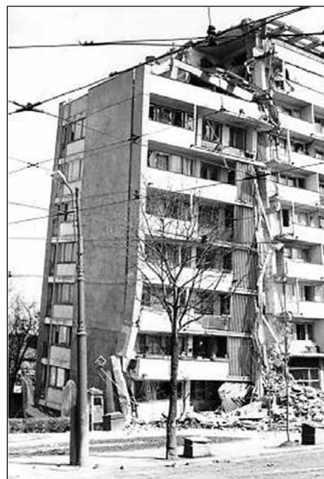
■ Foto 6. Blocul Lizeanu, colaps parter, 4 martie 1977 ■ Photo 6. Lizeanu Apartment Block, ground-floor collapse, March 4, 1977
