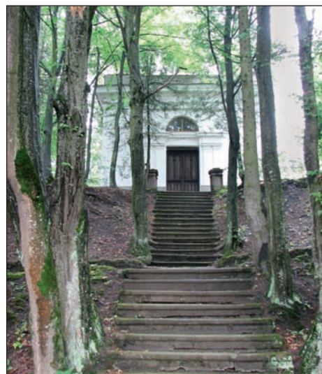
■ Photo 12. Alley with stone steps, climbing the slope towards the chapel. On both sides of the alley, trees are symmetrically placed, highlighting the steps' rhythm. The elevation with the entrance to the chapel forms the alley's upper perspective end, 2009 © Andreea MILEA
