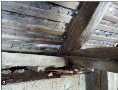
■ Table 2. Joint types of roof structure elements, Lutheran Church in Vurpăr and Toarcla
