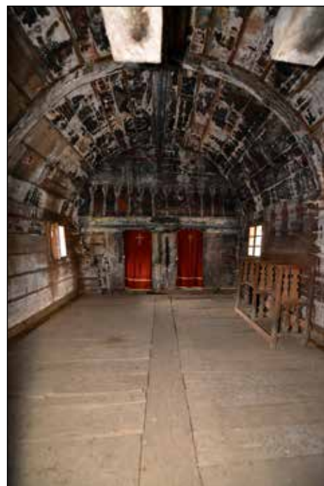
■ Photo 15. Calna, the naos with the vault supported by a single transversal arch © Ionel-Virgil POP
