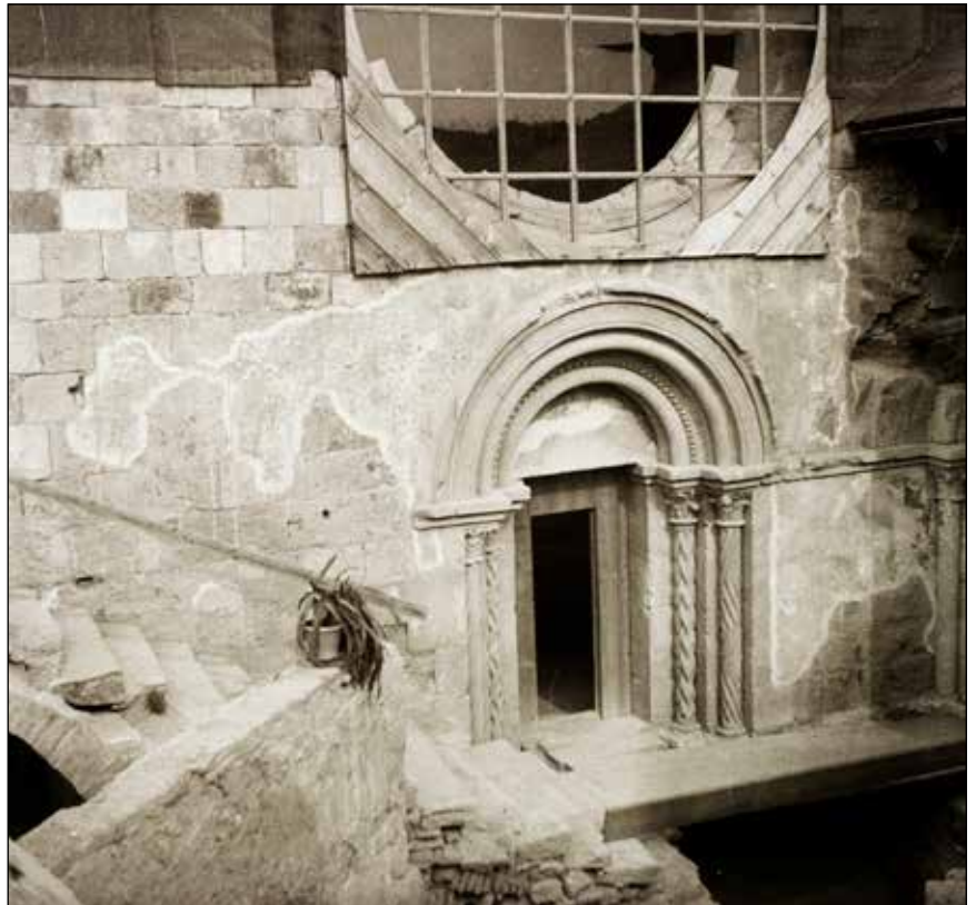
■ Photo 2. The entrance to the chapel of the Royal Palace of Esztergom in 1935, during the rehabilitation works © Fortepan, donator: Ebner (photo no. 83769, https://fortepan.hu/hu/photos/?id=83769 )
