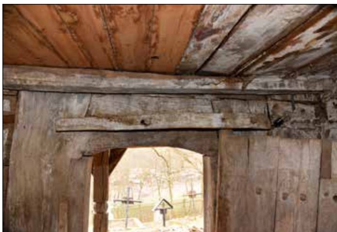
■ Photo 19. Calna, fitting method of the door with pintles and hanging stile made from a single piece of wood © Ionel-Virgil POP
