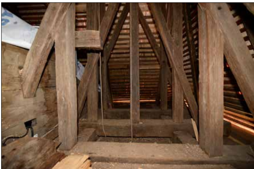
■ Photo 25. Calna, the lower part of the tower with oblique discharge into the beams that become stretched © Ionel-Virgil POP
