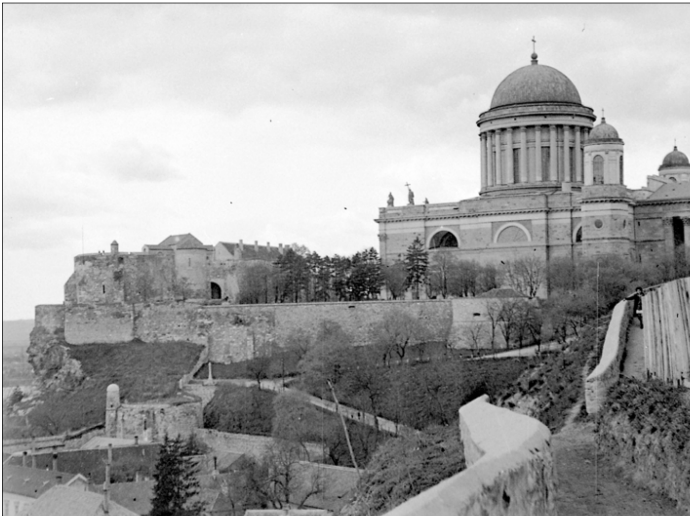
■ Photo 4. View of the rehabilitated palace from the east © Fortepan, donator: Fortepan (photo no. 2999, https://fortepan.hu/hu/photos/?id=2999 ) ■ Foto 4. Vedere a palatului reabilitat dinspre est © Fortepan, donator: Fortepan (nr. foto 2999, https://fortepan.hu/hu/photos/?id=2999 )
