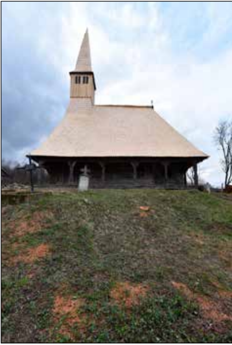
■ Photo 32. Calna, the south elevation, after replacing the shingle and clearing the terrain, 2021 © Ionel-Virgil POP
