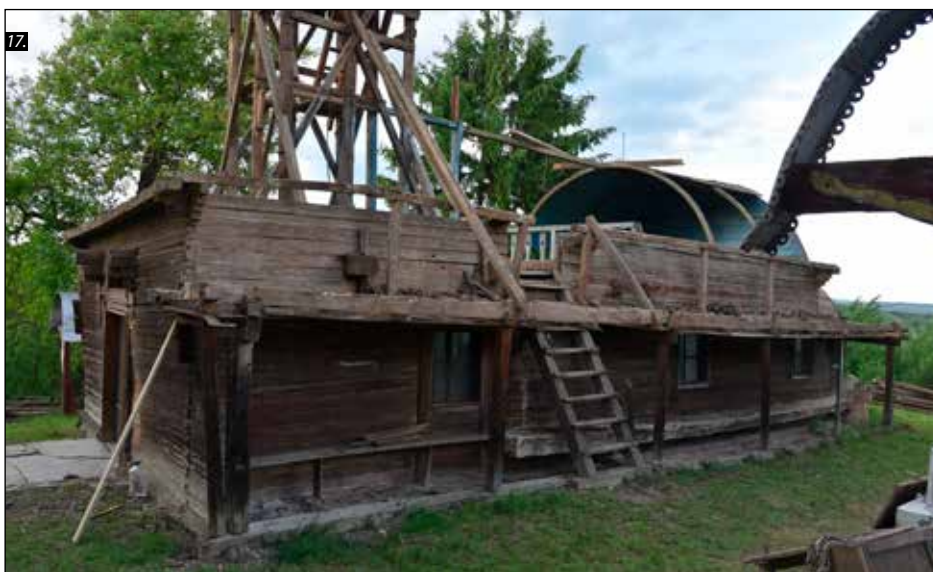
■ Photo 17. Cojocna (Cluj County), wooden church during conservation, note the gallery accessed directly from the pronaos © Ionel-Virgil POP
