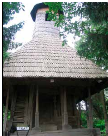
■ Photo 26. Pișteștii din Deal (Gorj County), the tower's posts reach the pronaos of the church © Ionel-Virgil POP
