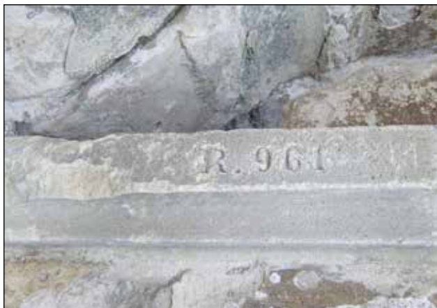
■ Photo 4. Carved stone replaced in the restoration with the inscription R 961 indicating the year of its replacement © Anna KINDE
