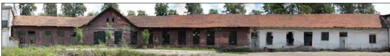
■ Photo 4. Mechanical Workshops photo © Tudor CONSTANTINESCU
