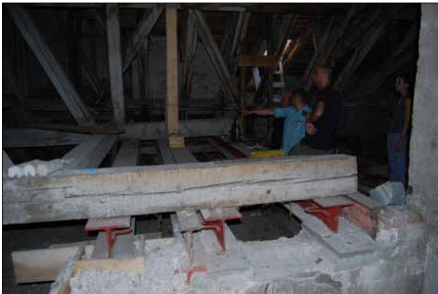
■ Foto 6. Intervenții de consolidare a șarpantei istorice © Bogdan DEMETRESCU ■ Photo 6. Consolidation interventions on the historic roof structure © Bogdan DEMETRESCU
