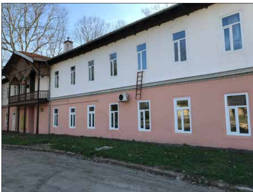
■ Foto 5. Fațada posterioară – detaliu tâmplărie PVC © bondstudio 2018 ■ Photo 5. The rear elevation – detail with PVC joineries © bondstudio 2018
