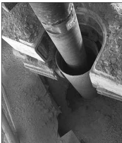
■ Photo 5. Drilling of the jacketed micropile
