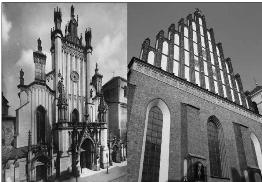
■ Photo 9. The façade of the Warsaw Cathedral before World War II and after the reconstruction The archival photograph's source (Biblioteka Cyfrowa Politechniki Warszawskiej); current state © Marek ŚWIDRAK
