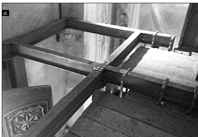
■ Photo 4. View of the bearing steel framework: a) from above and b) from below, with details of the hanging steel bracelets © Mariangela ROSSINO
