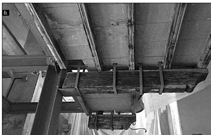
■ Photo 4. View of the bearing steel framework: a) from above and b) from below, with details of the hanging steel bracelets © Mariangela ROSSINO
