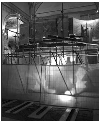
■ Photo 6. View of the moving scaffold supporting the choir loft
