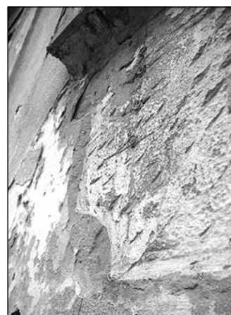
■ Photo 7. Imprint of the moulding discovered on the windows' apron, under the plaster (PESCAR, DRAȘCOVICI & ROȘIU 2017)
