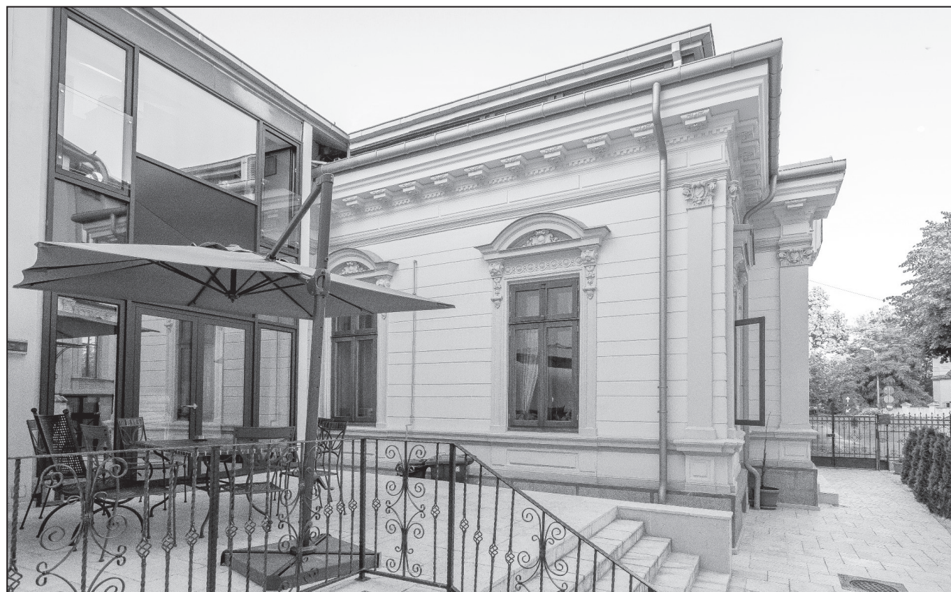
■ Photo 7. 17 Mântuleasa Street in Bucharest – the present condition of the southern elevation © Arthur ȚINȚU
