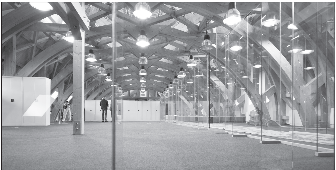
■ Photo 2. The Town Hall of the 1 st District in Bucharest – the new roof structure in 2015 © Gabriel CĂRSTEA
