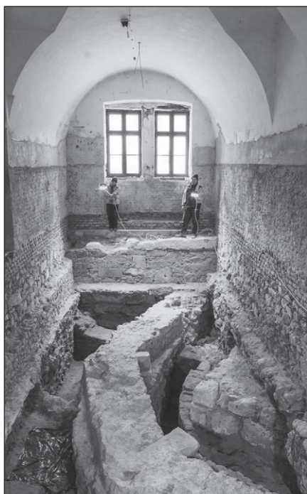
■ Foto 3. Fundațiile Bisericii Beata Maria Virgo minor, 2015 ■ Photo 3. The foundations of the Beata Maria Virgo minor Church, 2015
