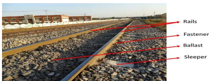
Figure 2 Railway components details
