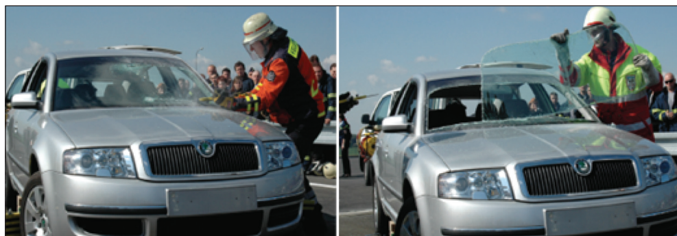
Fig. 3: Removal of windscreen with sawzall [8]
