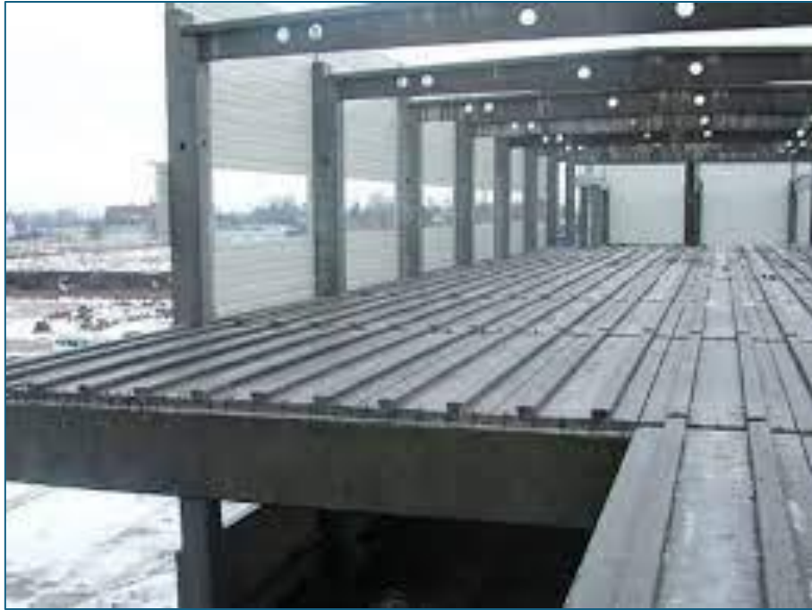
Figure 4: Top-ribbed formwork bark panel [5]
