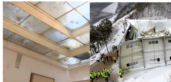
Fig. 3 Roof collapse due to the snow [ (a) Theatre in Czech Republic (b) University hall in South Korea]
