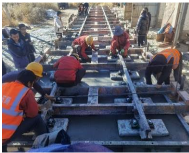
)a) Concrete pouring of ballastless track
