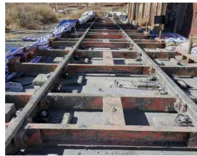
)b) Concrete maintenance of ballastless track
