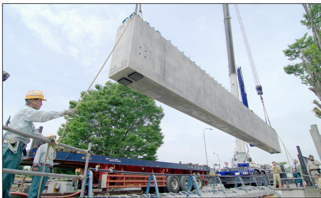
Fig. 20: Girder using zero cement concrete and aramid FRP tendons (2019)
