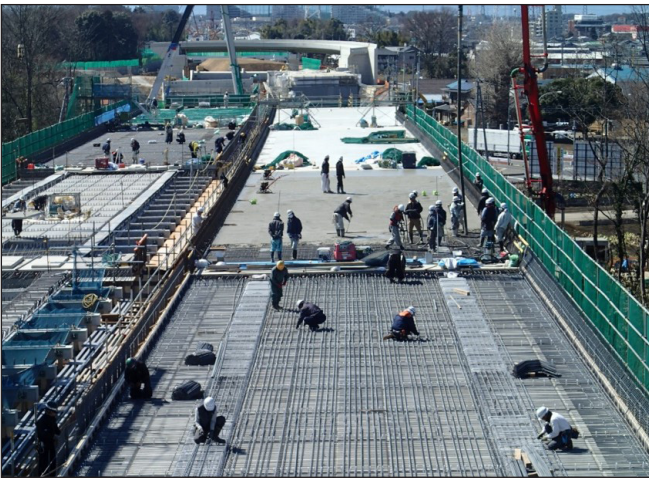
Fig. 9: Construction of cast-in-situ upper deck
