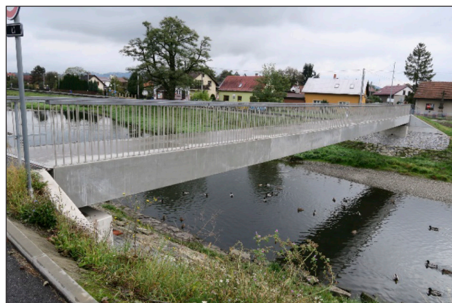
Fig. 20: Completed footbridge in Pribor (2019)
