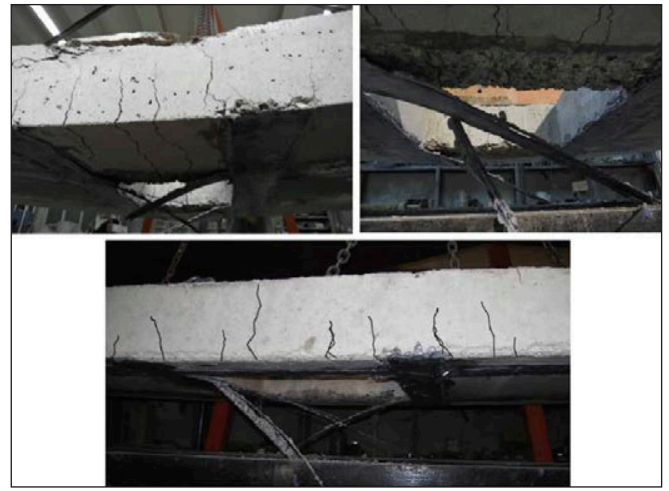
Fig. 7: Example pictures for CFRP failures
