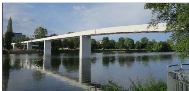
Fig. 25: A completed footbridge in Prague (2023)
