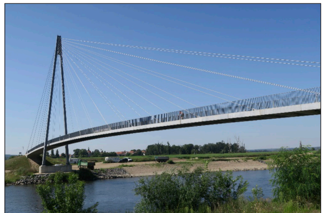
Fig. 18: Completed footbridge in Luzec (2020)
