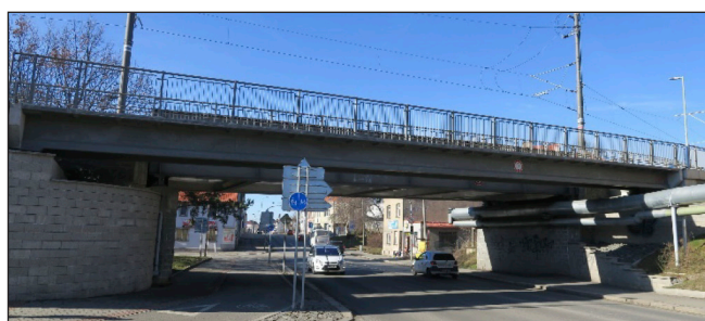
Fig. 22: Completed footbridge in Tabor (2018)
