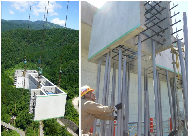
Fig. 4: Partial precast construction method for bridge piers
