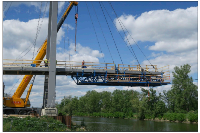
Fig. 17: Assembly of segments of the footbridge in Luzec
