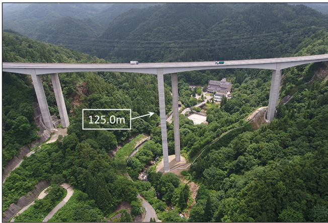
Fig. 3: The highest bridge pier In Japan
