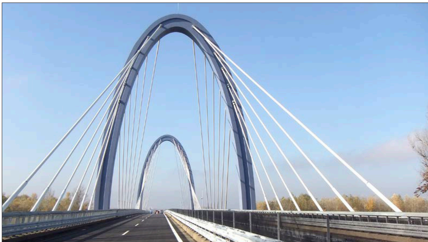
Fig. 7: View of the pylons from the bridge
