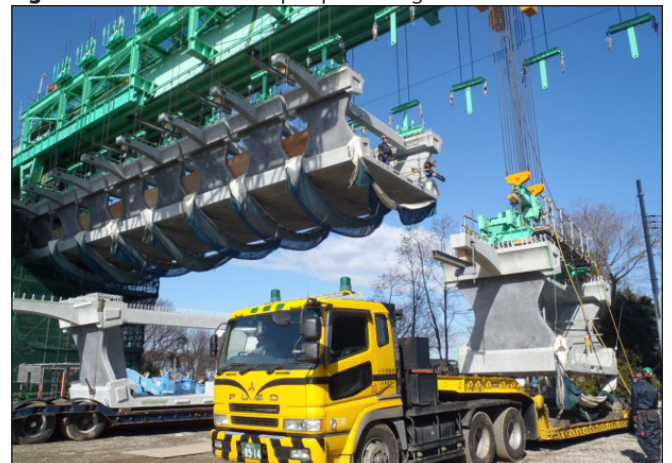
Fig. 8: Construction of U-shaped precast segments
