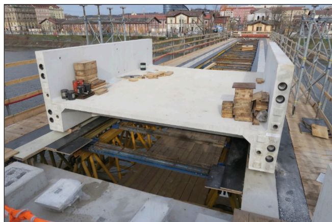
Fig. 24: Typical segment of the footbridge in Prague (2023)
