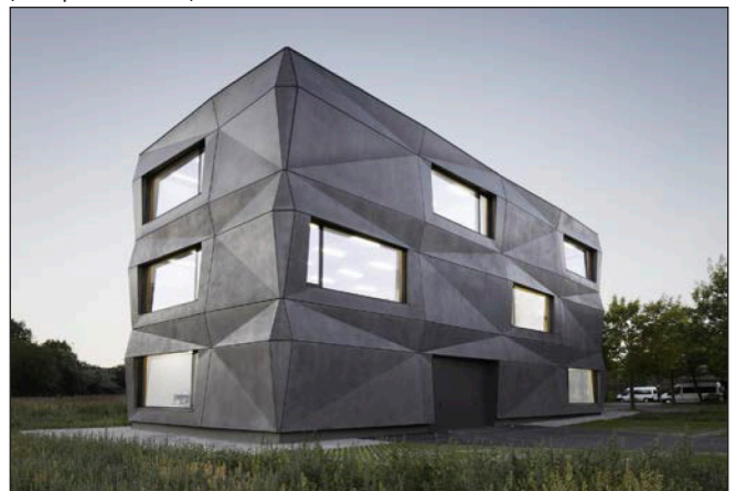
Fig. 13: Large-panel concrete facade, Designer: Tillicharchitektur (Compensis, 2013)
