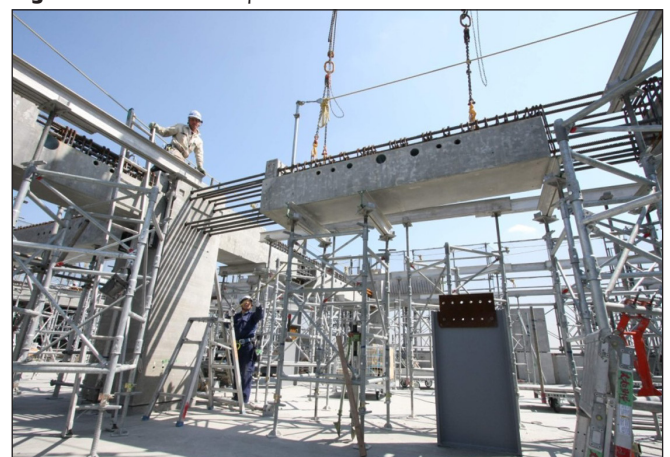
Fig. 2: Construction of a precast beam
