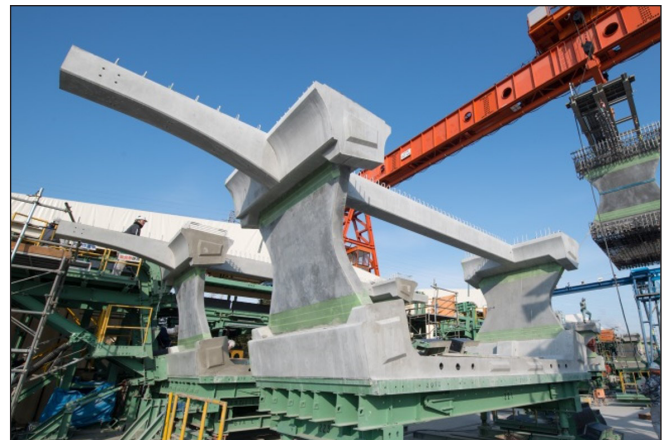
Fig. 7: U-shaped precast segment without upper deck
