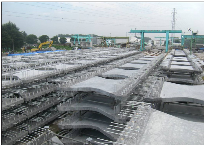
Fig. 6: Stock yard of butterfly web panels
