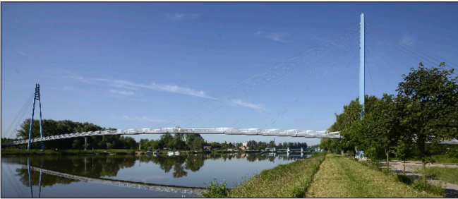
Fig. 15: Completed footbridge in Celakovice (2014)
