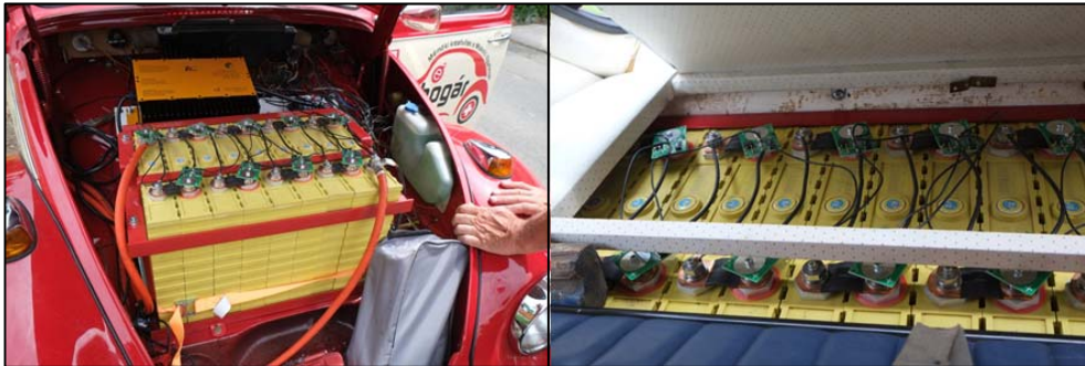
Figure 2. 9 LiFeYPO 4 batteries in the trunk (left); 15 cells behind the rear seats (left)
