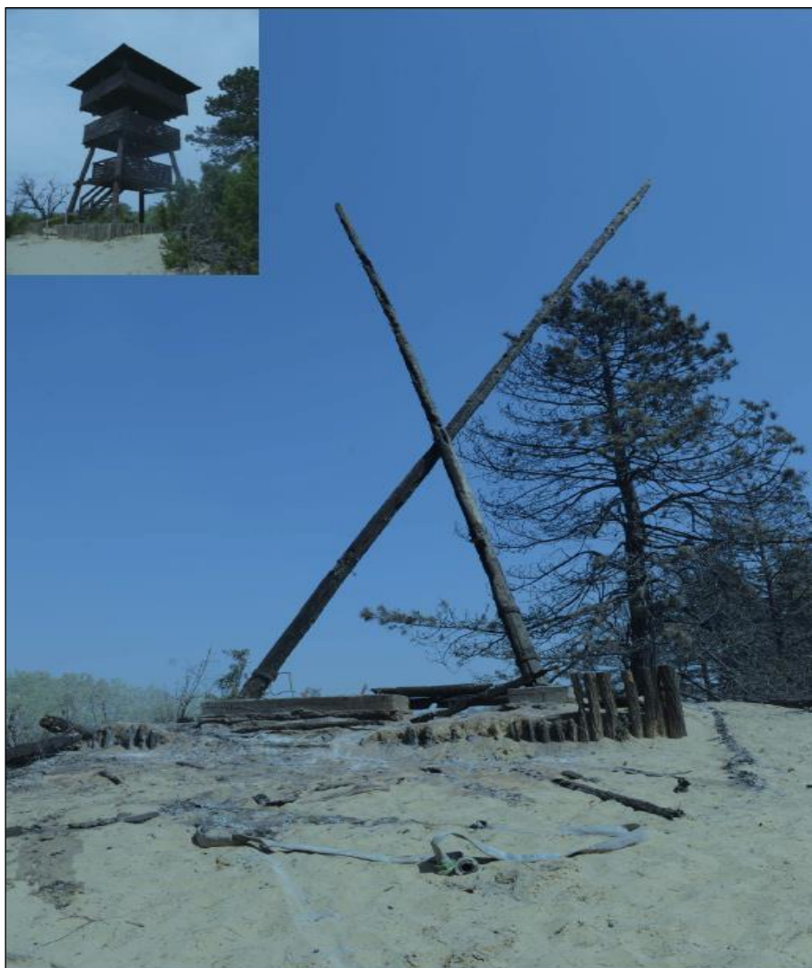
Figure 15.: Destroyed observation tower, burnt firefighting equipment in Bugac (Source: [18])
