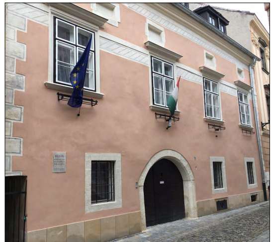
Figure 5. The restored street-facing façade of 8 Új street. (author's photograph)
