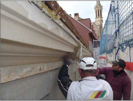
Figure 2. Moulding the fascia of the St. György street façade of 2 Hátsókapu, using a mould knife (author's photograph).
