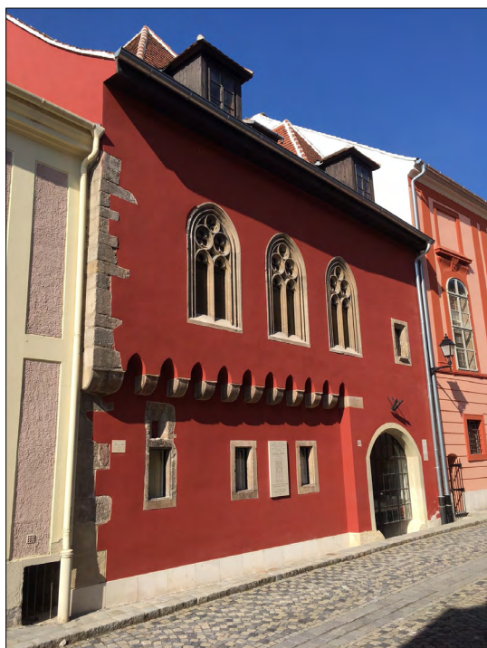
Figure 4. The restored street-facing façade of 16 Új street (author's photograph)
