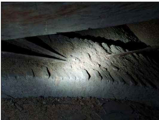
Figure 3. The tie rods connecting the walls, the vaults and the roof structure.
