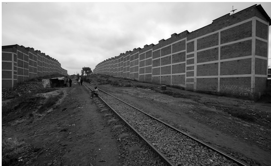
▲ Photo 6. New residential buildings, apartments in Kibera were erected in the frame of the KENSUP project. Own photo.
