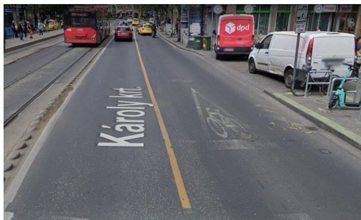
Figure 7. – Bottleneck near Astoria square, worn road signs source: Google Street View https://goo.gl/maps/kLoUSSGHPnz9CQBN9
