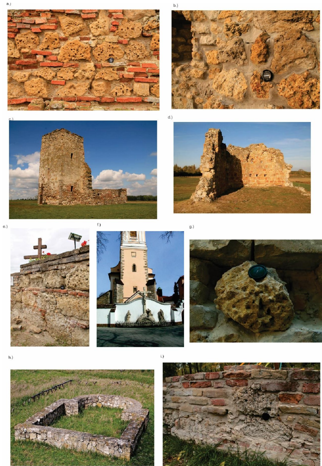
Fig. 1.: Medieval church walls and church foundations built of freshwater limestone of the Danube-Tisza Interfluve, Hungary
