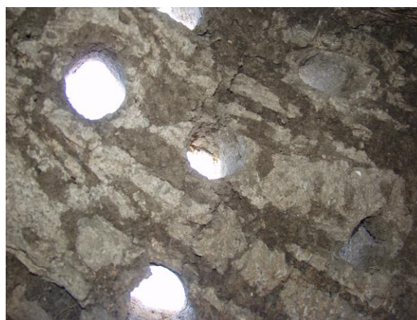
Fig. 7.: "Smoke tunnels" on the kiln's raised floor
