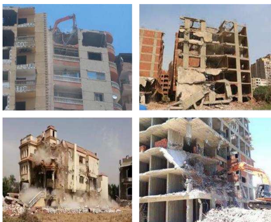
Figure 2. Examples of Demolishing Buildings [25]
