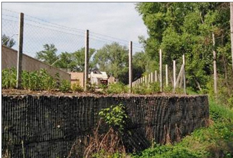
Picture 6: The North side of the WWTP
