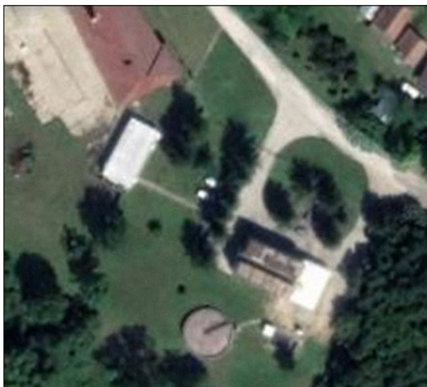
Picture 7: Top-view of the WWTP
