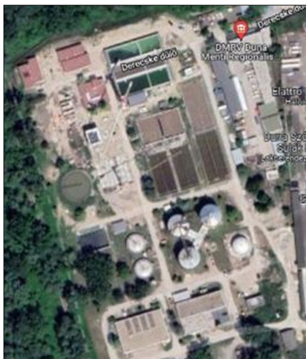
Picture 5: Top-view of the WWTP
