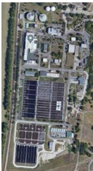
Picture 1: Top-view of the sewage treatment plant
