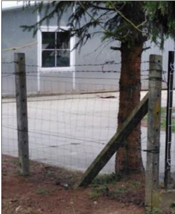
Picture 9: One element of the fence on the northern section of the WWTP
