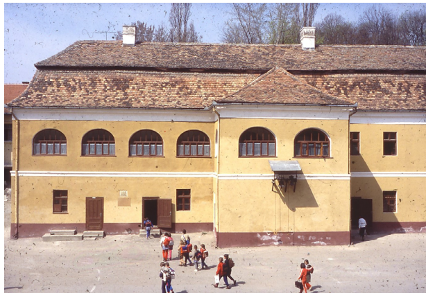
Figure 1. The Building of the Bethlen College in Nagyenyed
