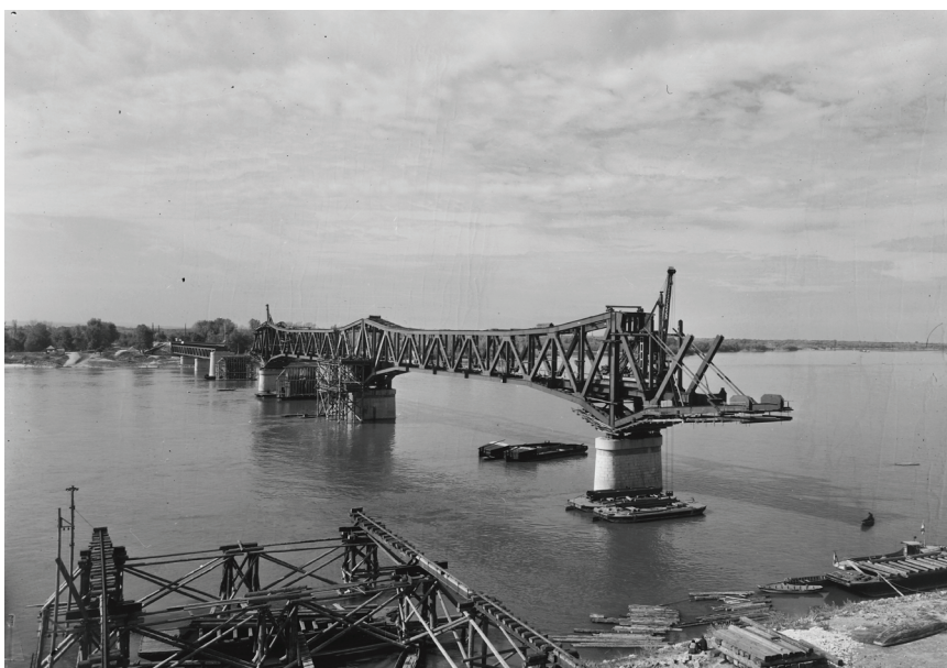
Picture 2. Rebuilding the Danube-bridge in Baja, 1950. (Fortepan, No. 91383)
