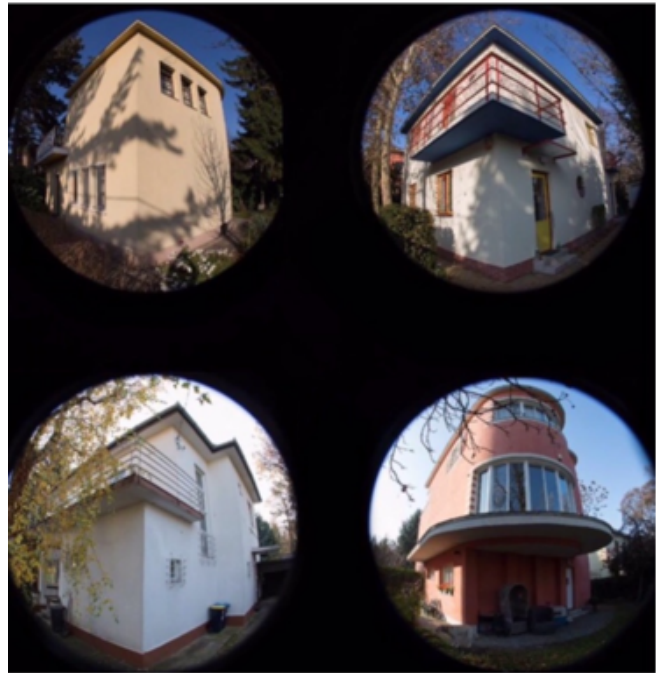
Fig. 12. Some of the houses of a group of villas, influenced by Farkas Molnár, and other works from the Bauhaus. They were quite similar to the contemporary Weisenhof Siedlung in Germany – at the time and in the same location, around the early Thirties
