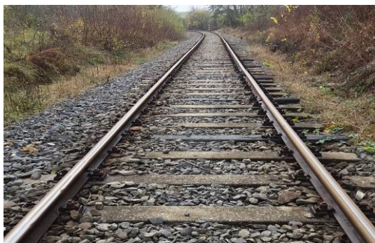
Figure 5. Railway superstructure of the tested section
