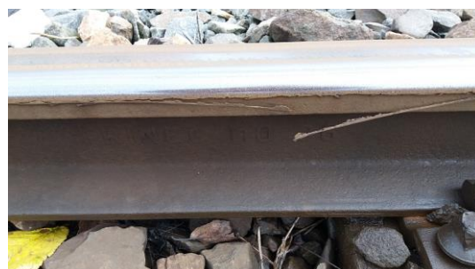
Figure 8. Lip on the rail head
