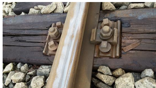
Figure 7. Pushed baseplate
