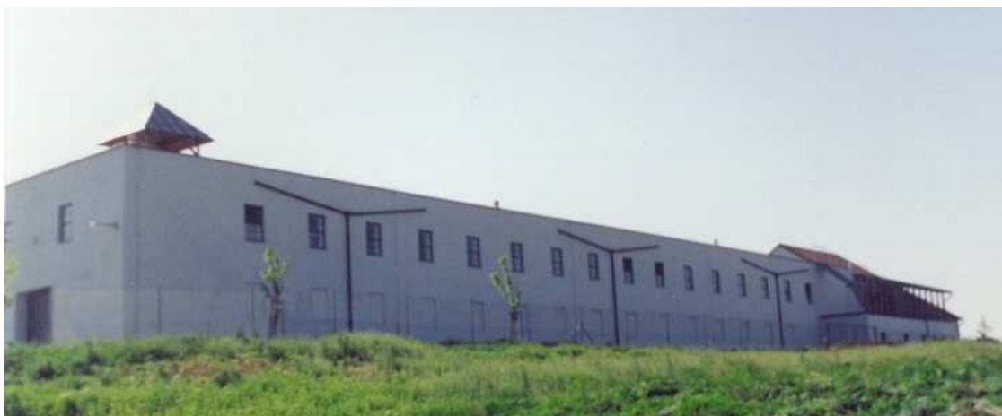
Figure 4 State of a new production and storage hall with name ‘ Mlaty ’ after first reconstructions in 2001
