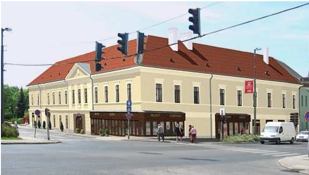
Figure 5: Restored historical building int he walking street
