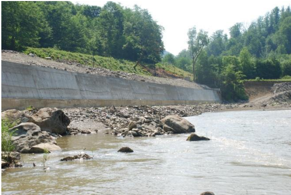
Figure 8. Vișeu River banks anthropogenic modifications
