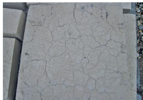
Fig. 7. Map-like cracks
