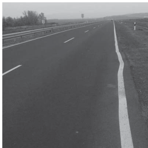
Fig. 2. Because of the build in tissue net, the abrasion layer slipped and a rut has appeared (route 21.)
